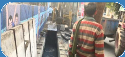
The authority is conducting drainage cleaning work
